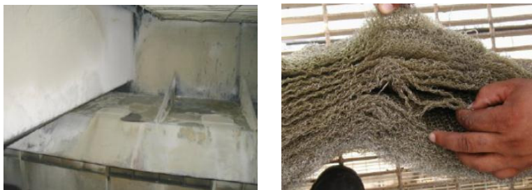
Figure 5.36: Slight dusting deposits in the flashing chamber and on demisters
