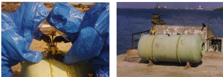
Figure 9.5: The installation of the special designed hood assembly
