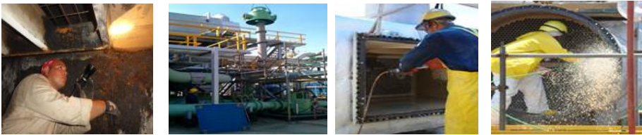
5. Internal inspection 6. Brine pump removal 7. Hydrolase long tubes 8. Brine heater cleaning
