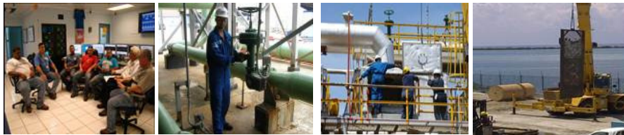
1. Pre GI- meeting 2. External Inspection 3.Vessel cover removal 4. Intake screen removal
