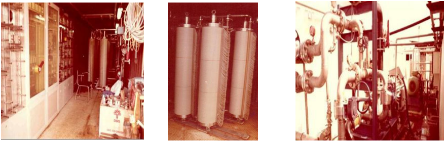
Membrane Section Plate and frame membrane High pressure pump section
