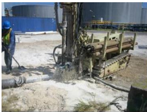
Figure 10.7: Drilling of beach wells at W.E.B. Aruba N.V.
