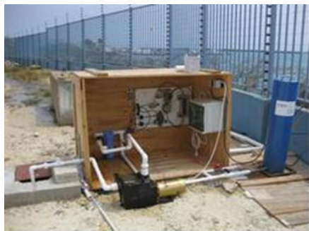
a: provisional beach well monitoring
