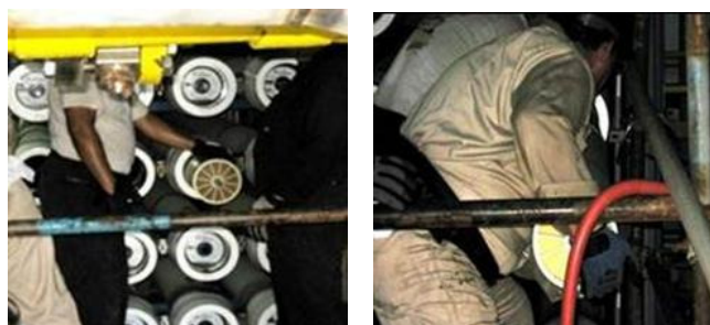
Figure 8.11: The membrane changing activity at the Desalination Department
