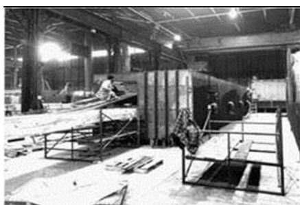
a: Copper tubes installation in MSF vessel
