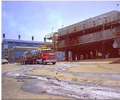
b: acid spill and corroded vessel
