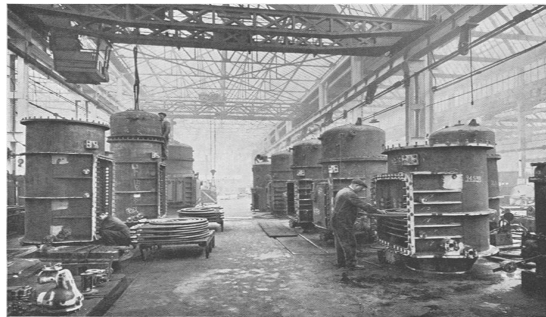
Figure 2.25: The construction of single stage evaporators at WEIR Inc. around 1912 [2.5]
