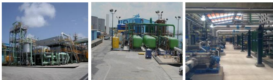
MSF Technology: 6,000 m 3 /d SWRO Technology: 8,000 m 3 /d SWRO technology: 24,000 m 3 /d Aqua Chem Inc. GE WPT Veolia VWS
