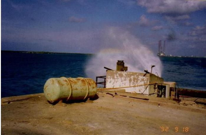
Figure 9.6: The chlorine disposal system with the seawater curtain
