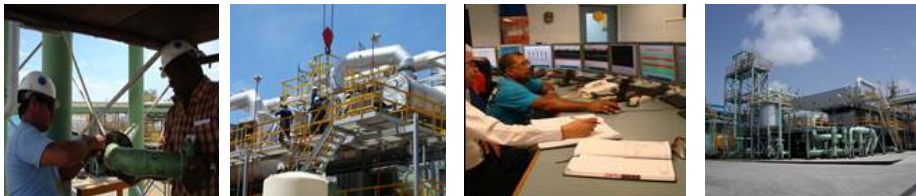
9. Repair vacuum pipe 10. Closing vessels 11. Performance post GI 12. Plant in Operation
